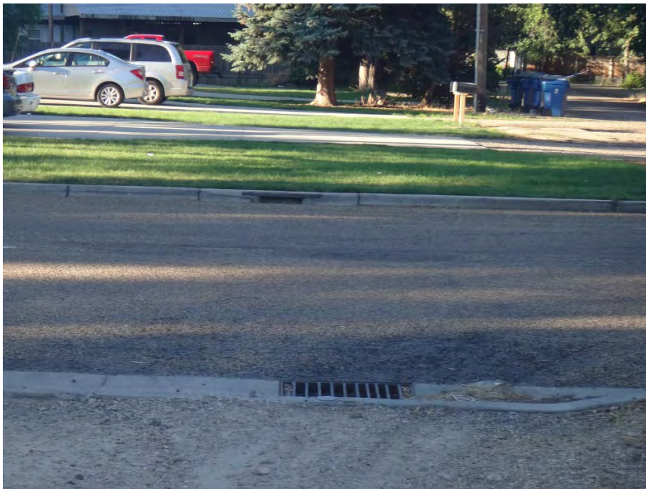
Figure 7: Outfall MS-1.170 Catch Basins
