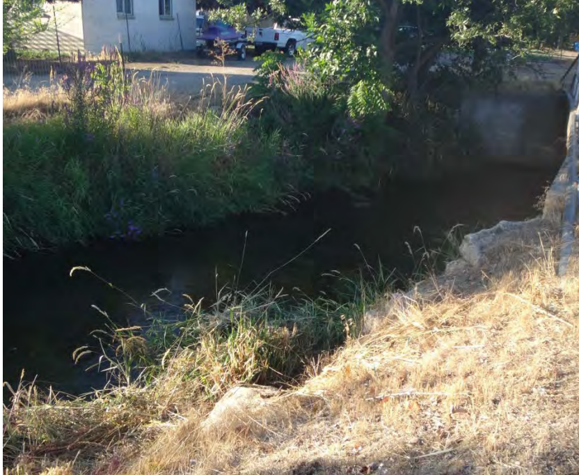
Figure 9: Outfall MS-1.180 location on canal bank
