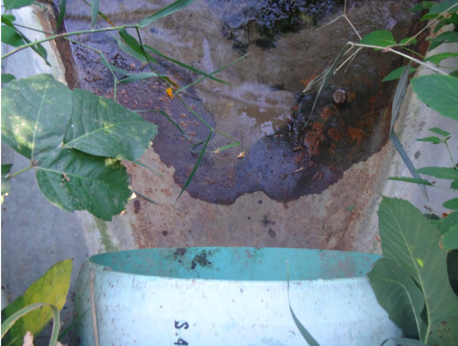
Figure 11: Outfall LK-1.10 flow indicator
